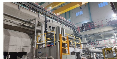
Sulfuric Acid Production and Waste Heat Power Generation Expansion Project
