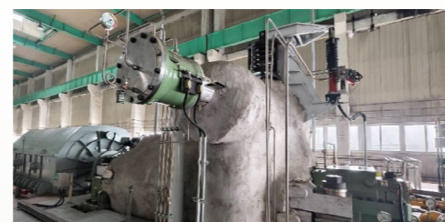
Steam Turbine Retrofit Project
