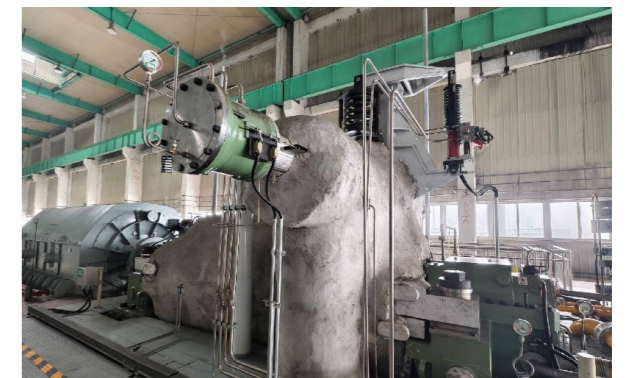
Heating Station Water Pump Renovation Project
