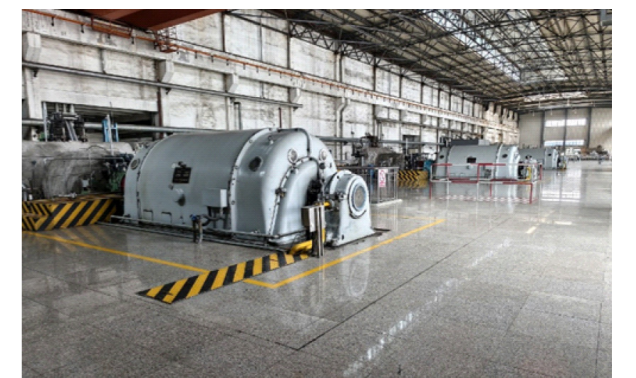
High-Efficiency Boiler Upgrade Project
