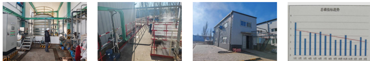
Technical Upgrading of Wastewater Treatment Workshop
