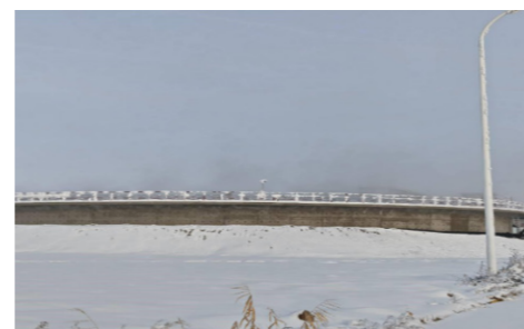
On-Site Photo of The Pretreatment Facilities
